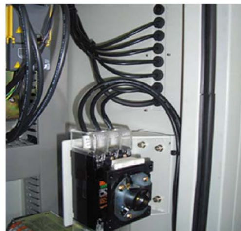
Rubber seals are mounted at the EC cabinet door for optimal enclosure.
